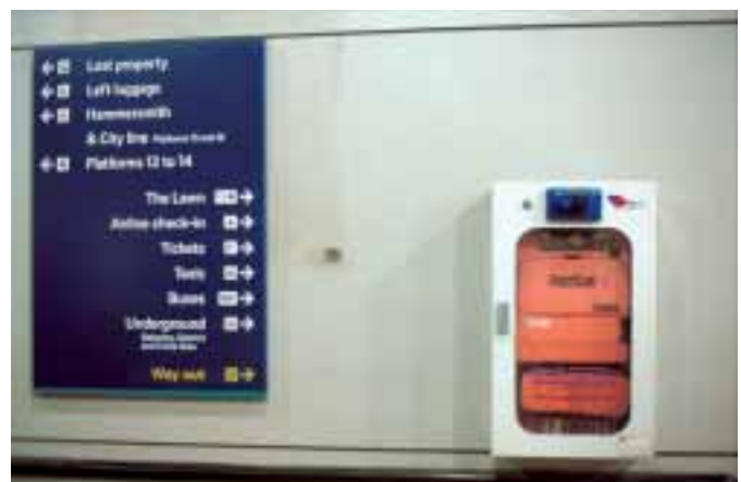
AED on a railway station
