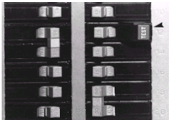
Figure 8-29. Special GFCI circuit breaker. The arrowhead points to the distinguishing red test button.
