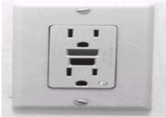
Figure 8-28. A ground fault circuit interrupter (GFCI) electrical outlet with integrated test and reset buttons.
